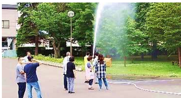
Demonstration of fire hydrant: pressure of the water discharge was strong and sprayed quite high
